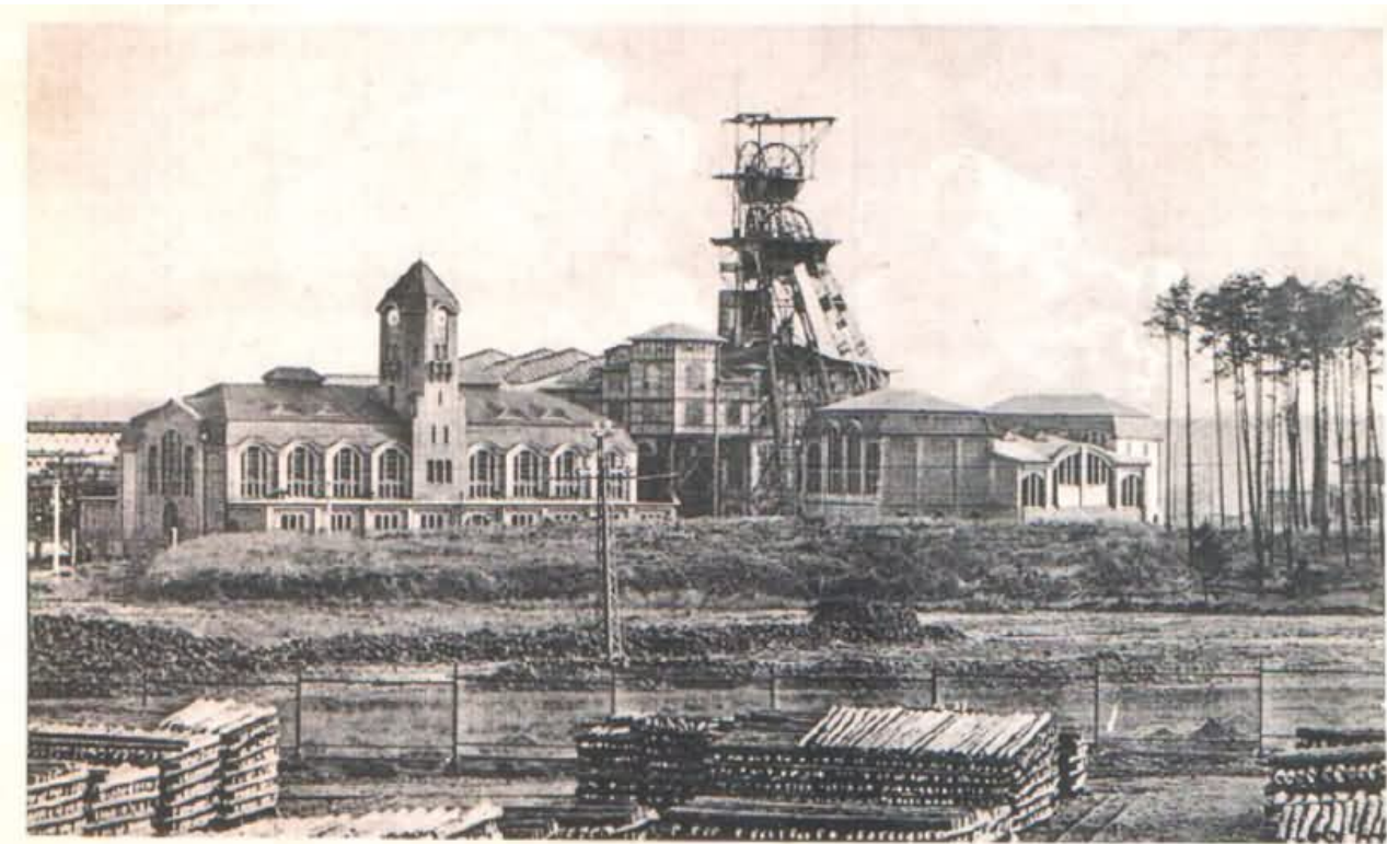
GIESCHE-GRUBE — Carmar Schacht
